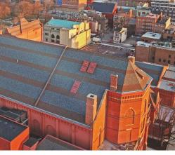
The vents were installed above the main hall, Springer Auditorium, and are designed to open in an emergency to allow smoke and hot gases to escape. This allows better visibility and breathing conditions for audience members and performers to evacuate safely and aide firefighters in their containment efforts.
