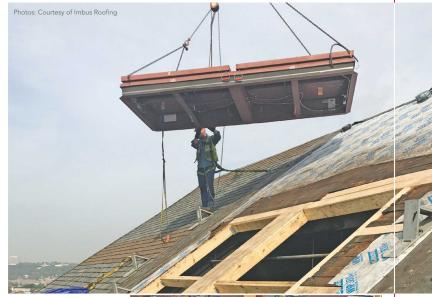
The vents are hard-wired to the fire suppression system and open electronically if the sprinkler system activates. Corken Steel, the local distributor of the smoke vents, and BILCO rep Joe DeFrain of Welling, Inc., worked with Imbus in procuring the roof hatches.
