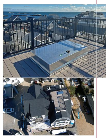
and cover design that minimizes heat transfer between interior and exterior metal surfaces delivers year-round energy efficiency.
