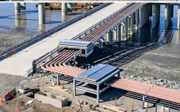
of Haskell Corporation, a mechanical and structural subcontractor. "The hatches also allow access to the expansion joints should they need to be replaced."
