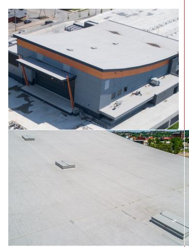
Double leaf automatic smoke vents are the most economical way to add fire venting protection in large areas, and are available in steel or aluminum construction. The curb-mounted fusible link housing allows the latch to be quickly and easily re-set from the roof level.
