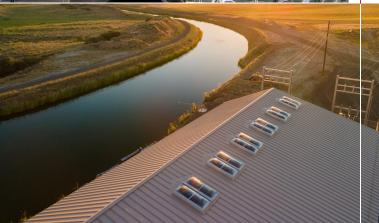
Teams will access the pumps through roof hatches manufactured by The BILCO Company. The custom hatches are fabricated with polycarbonate dome covers for natural daylight and engineered lift assistance for easy, one-hand operation. They are also modified for hand winch operation, allowing them to be easily opened and closed from inside the building.
