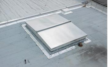
radiation source as necessary, without having to remove the equipment. "They will have to replenish the radiation source by going in through the roof, so this hatch allows them access to do that," Kersten said. "There isn't any other way to do that."
