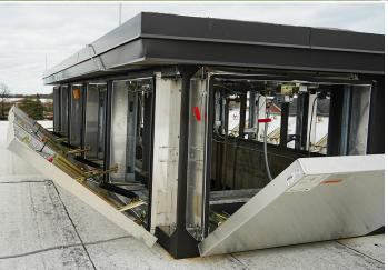
Smoke vents play an important role in helping firefighters bring a blaze under control. They protect property and aid firefighters in bringing a fire under control by removing smoke, heat, and gases from a burning building.
