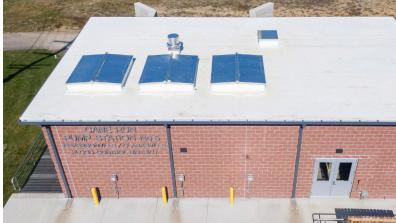
The project includes three roof hatches for access to the vertical turbine pumps, two floor doors that lead to a lower trough and a LadderUP safety post. Midwest Metal Works provided the doors for the project through BILCO's distributor in the region, Welling Inc.
